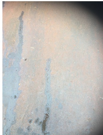
Steel plate covered in rust.
