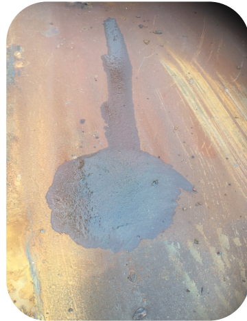
HENCO 1010 applied; 5-10 min waiting time and then agitated with medium hard bristle brush.
