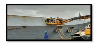
This shows our launch product, HENCO 1010 being applied with a medium-hard brush before being rinsed off with water after 10-15 minutes
